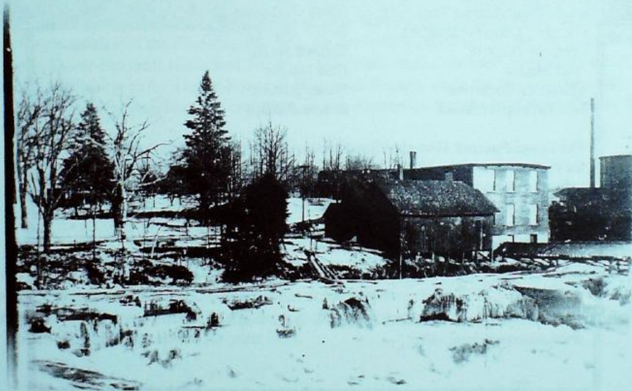
A view of Brown's Woolen Mill ca. 1900, where many people named in the 1904 Town Register worked. For more on where people worked in 1904, see page 1.
