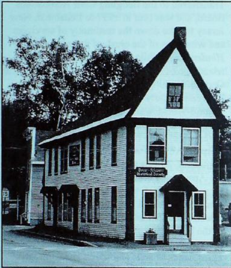
The restored facade returned the Observer Building to its look from the late nineteenth century. Photo by Jack Battick.
