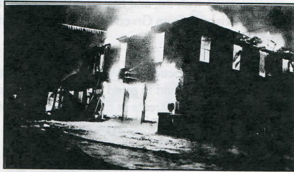
Flames engulfed the restaurant and shops nearest to the bridge. Photo courtesy of Alan Smith.
