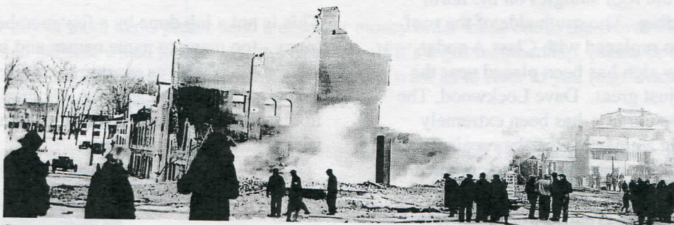
Spectators in Monument Square gaze at the ruined Opera House. The Masonic Building is at the rear right in this picture. Photo Courtesy of Alan Smith.
